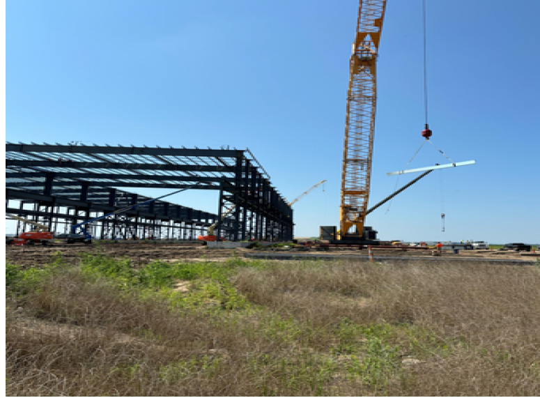
Steel Erection
