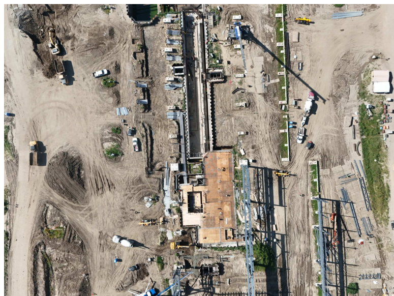
Aerial Photo - Rolling Mill Basem
