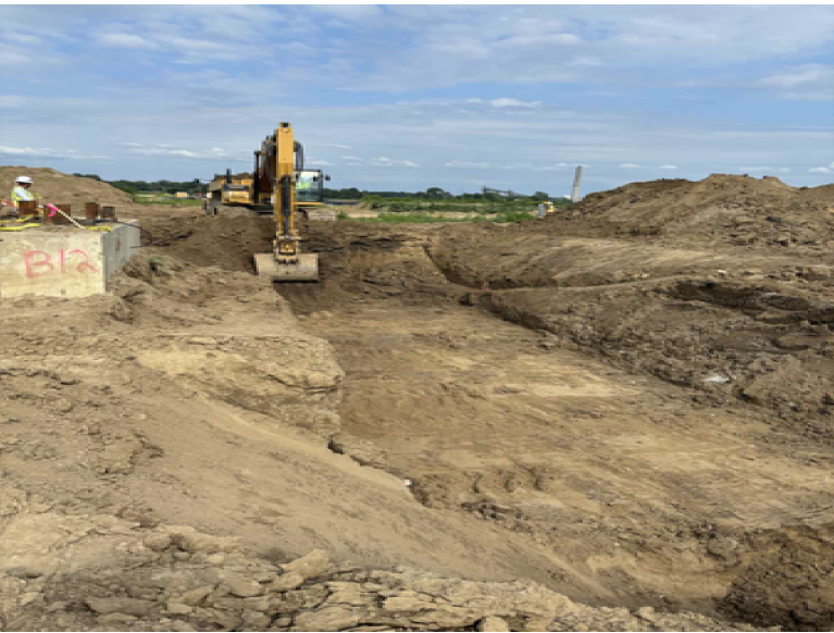
Underground Pipe Trench Excavation
