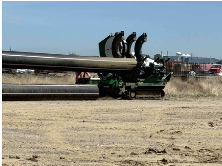
Underground Pipe Fabrication
