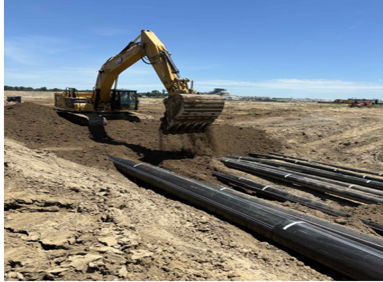
Underground Pipe Installation
